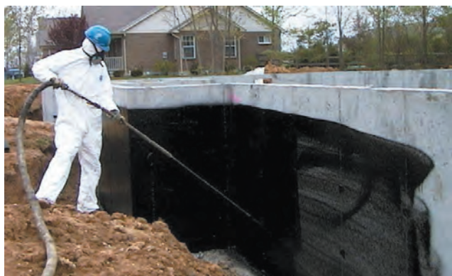
A basement stays dry with J-Cote™ WB by forming a seamless barrier that stops water even if the basement cracks.
