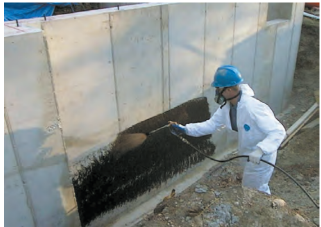
When installed by a Professional Selected Contractor, Hydra-Guard™ WB will provide years of worry free protection from water seepage.
